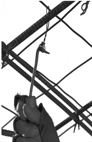
Tying off welded wire mesh.
