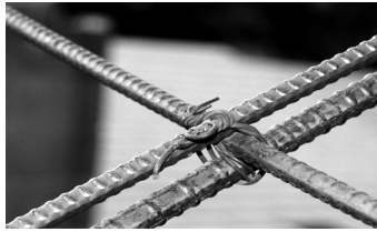
Double rebar tied.
