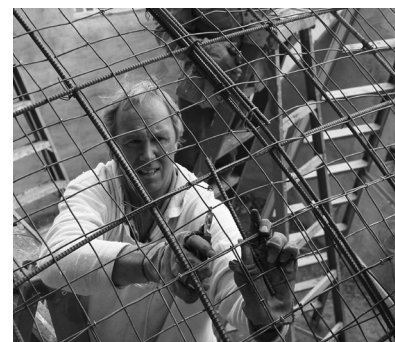
Tying off welded wire mesh with hog ring pliers.
